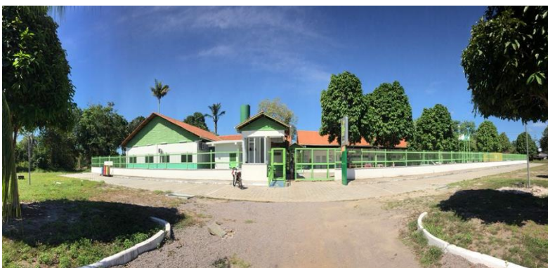
Figura 6 – Fachada principal do Campus
